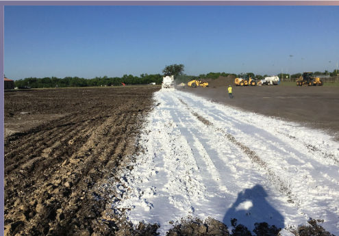
Moreno JHS - Lime Stabilization_05.21.2018
