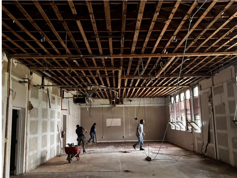
Main Building - Office Upgrade
