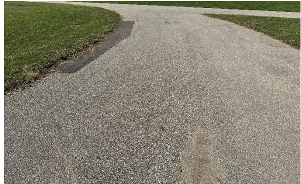
Photo 2: Surface Deformation – North Curve
