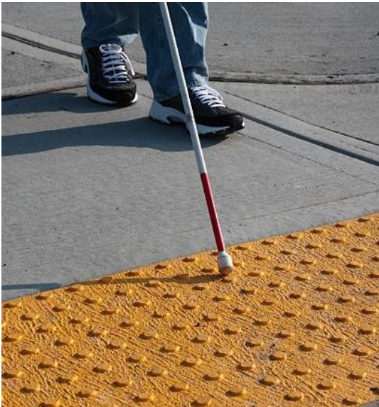
Truncated Dome Warning Devices
