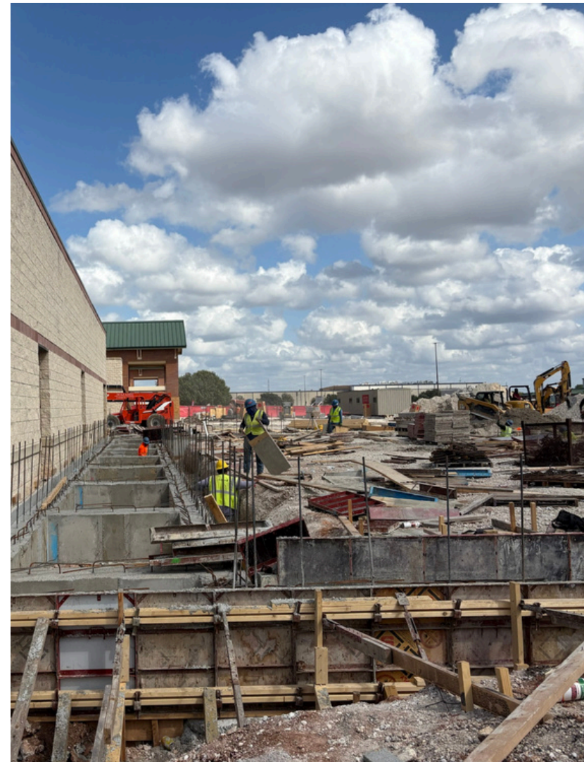
Completed Grade Beams
