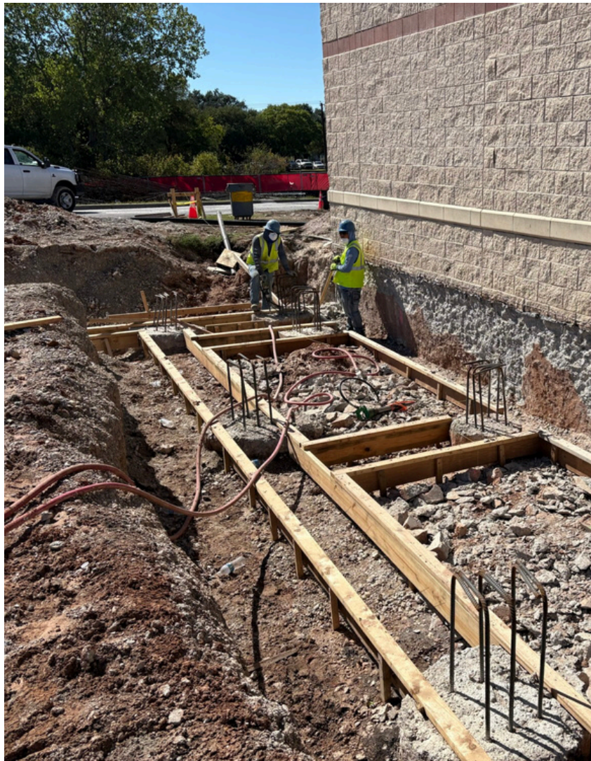
Forming Up Grade Beams
