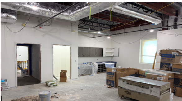
CLASSROOM w/CASEWORK MOCKUP
