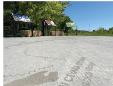
Example of sidewalk sandblasting: Richard T. Anderson Conservation Area in Eden Prairie, MN.
