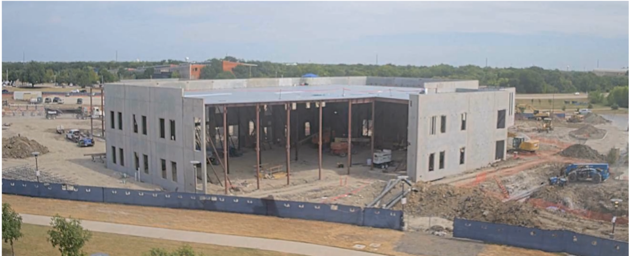
Tilt Wall Panels Erected, Roof Deck In Progress
