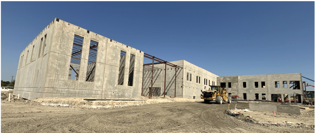
From the Southeast - Welding Bays, 2 Story Admin & Classrooms, 2 Story HVAC Wing
