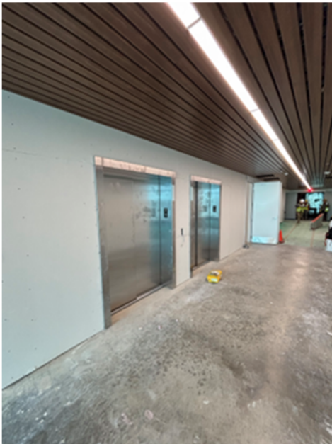
Level 1 Elevator Lobby
