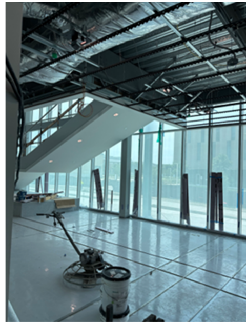
Level 1 – West Lobby Terrazzo Install
