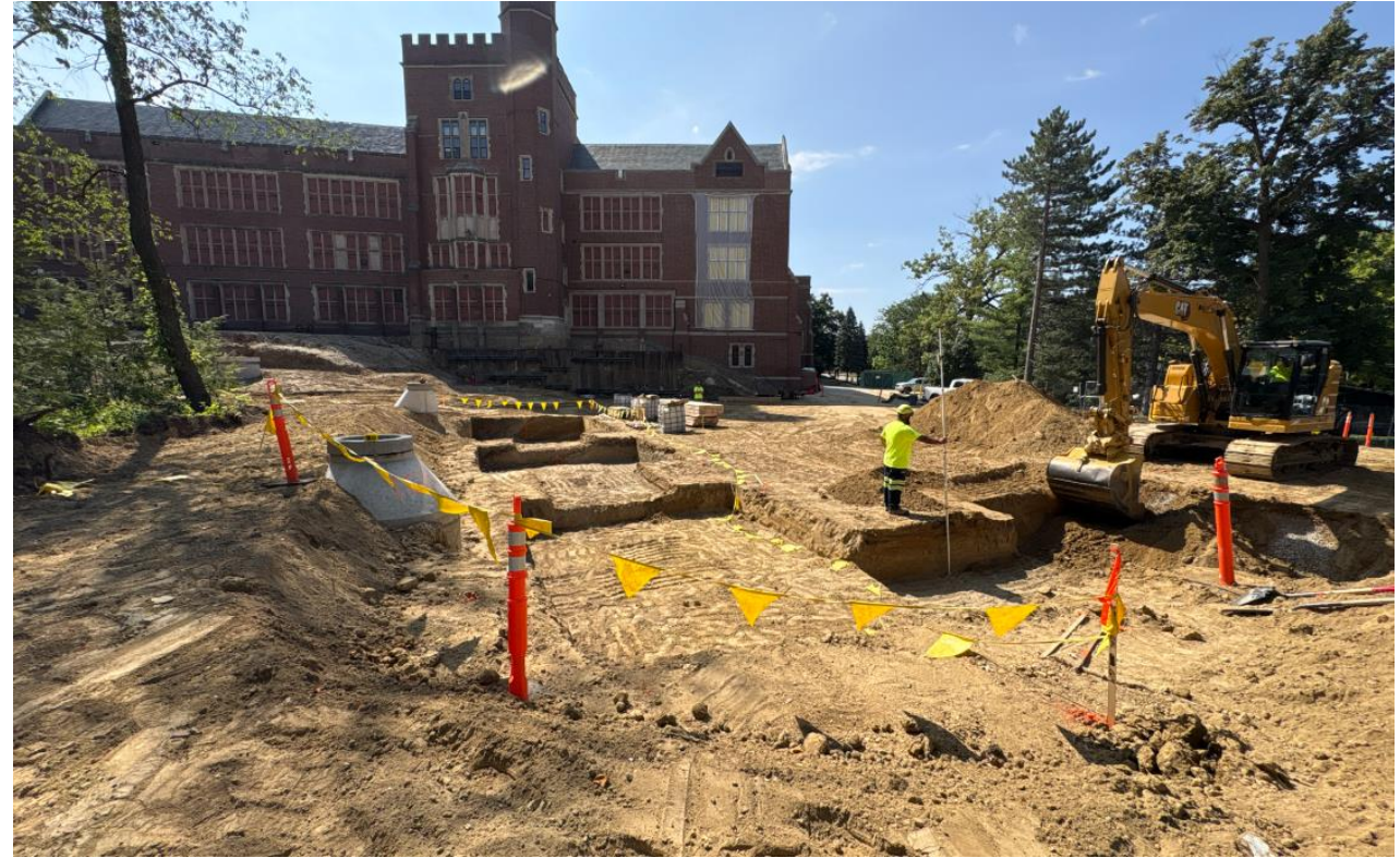
Classroom Wing Footings In Progress
