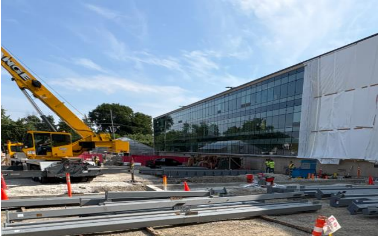
West Curtainwall Replacement
