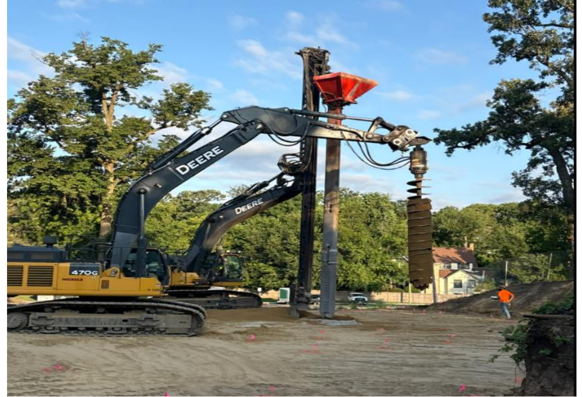
Rammed Aggregate Piers Installed
