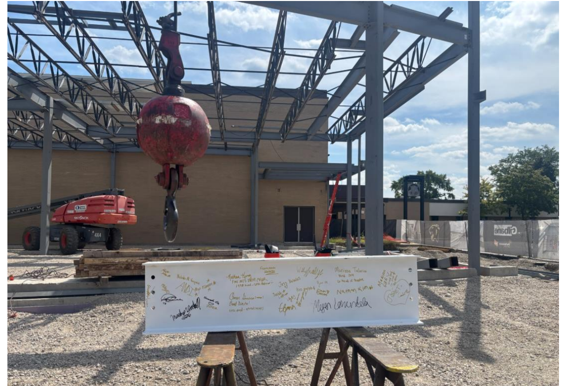
Music Addition Structure Topped Out
