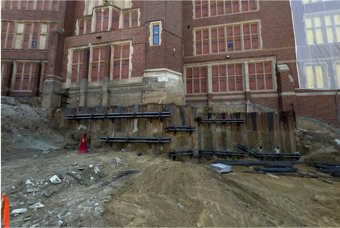
Earth Retention System Complete
