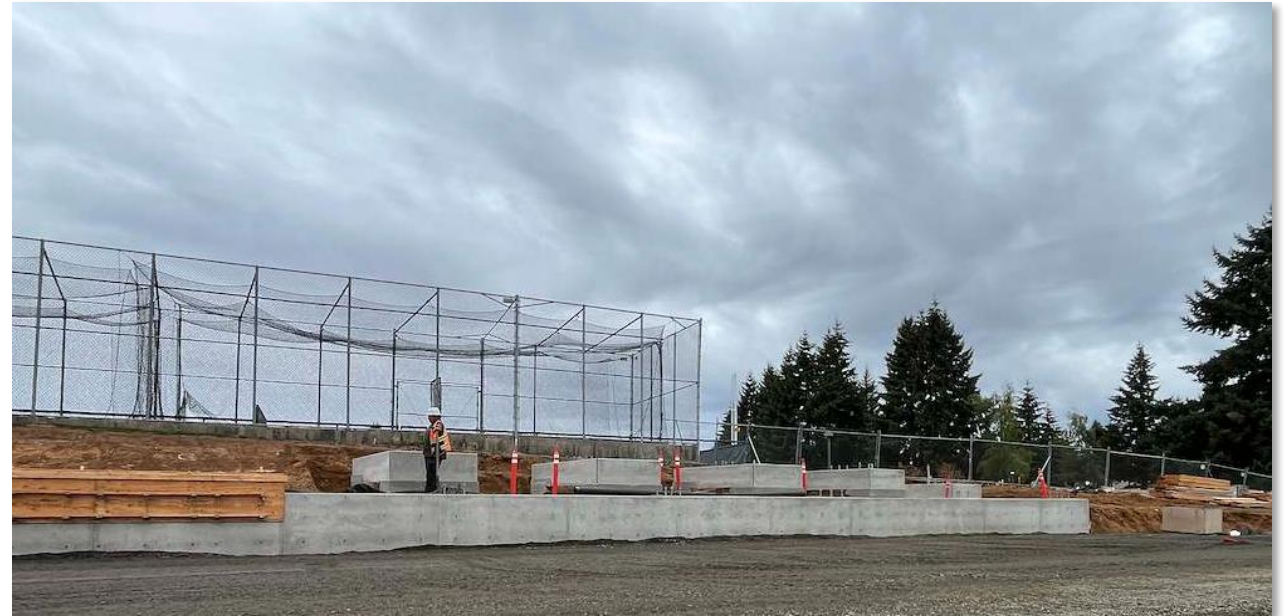
Massive Footings for Grandstand Roof
