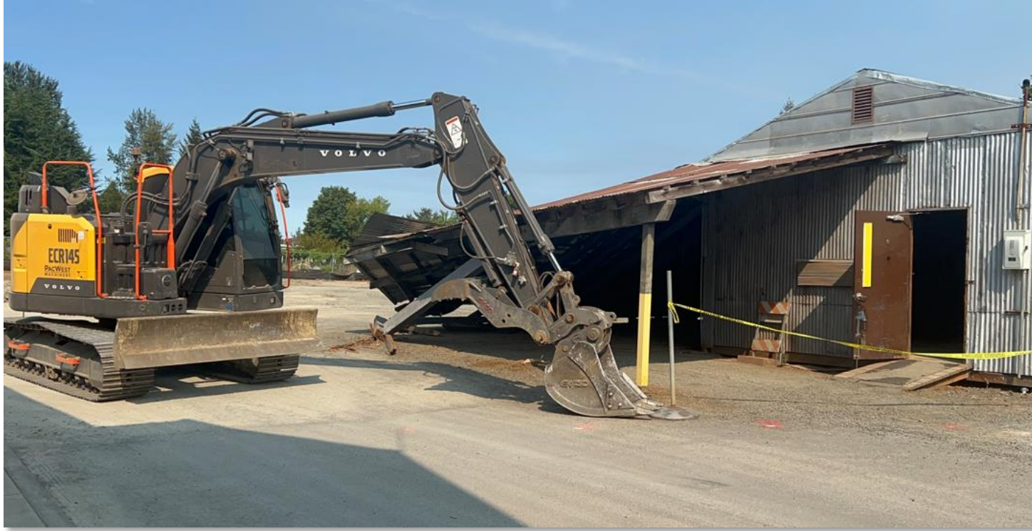
Demolition of the Campus Services Wood Shop
