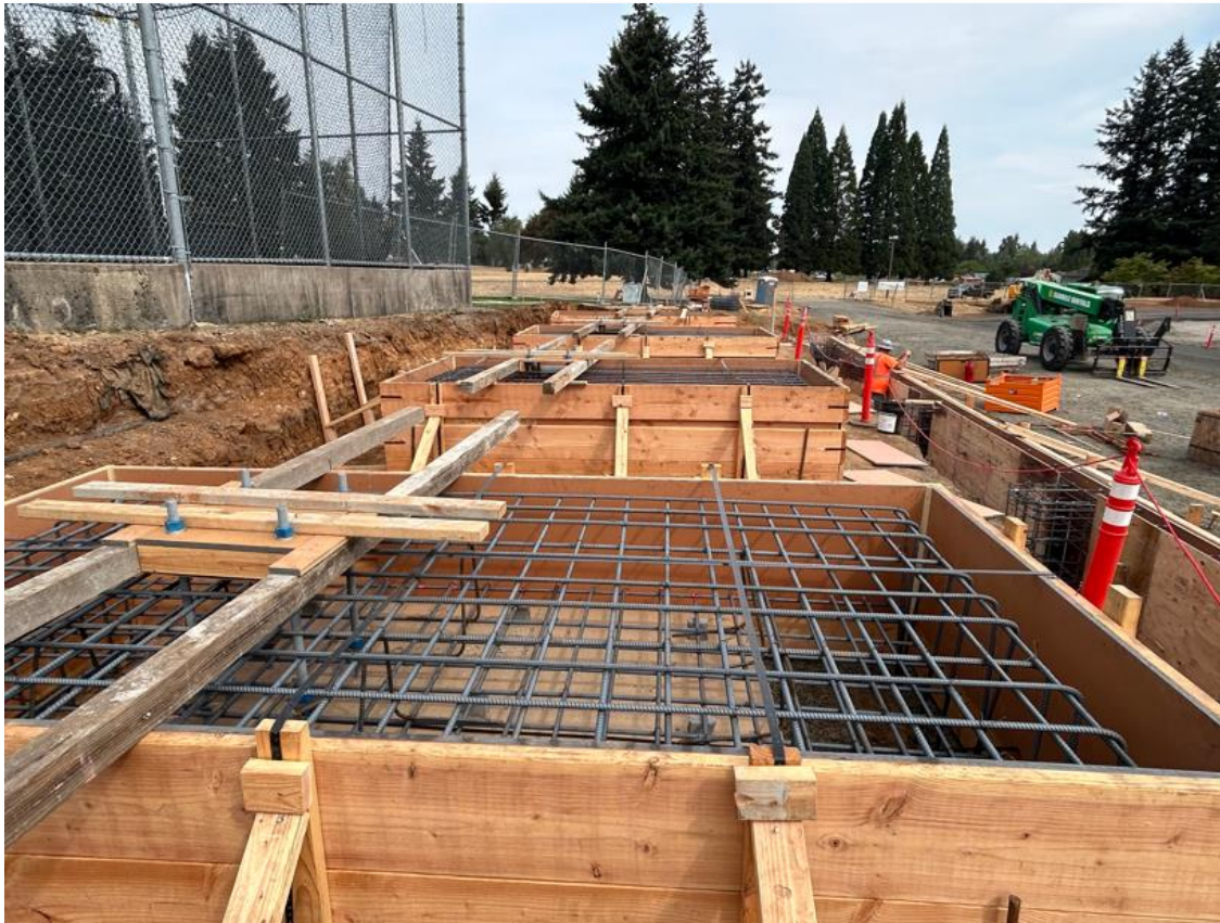
Massive Footings for Grandstand Roof
