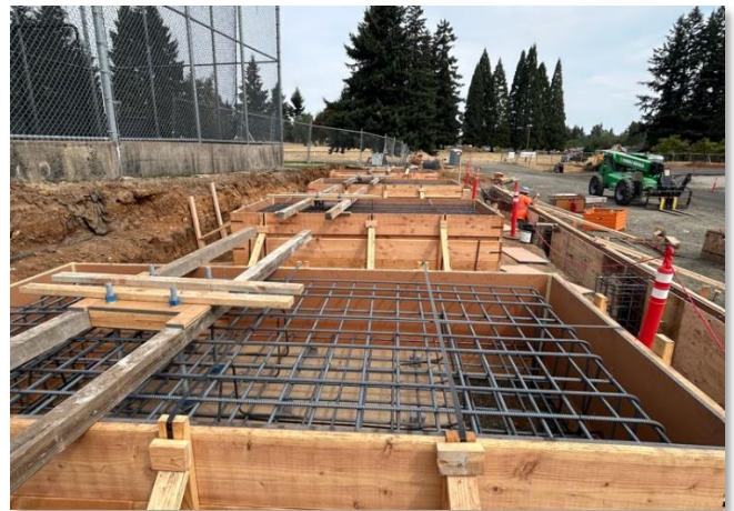
Large Footings for the Emerging Grandstands.
