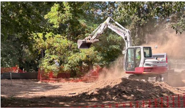
Maintenance Yard Project has Started. New Drainage Swale on Left, Cleared Yard on Right.
