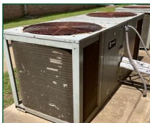
End-of-life condensing units & equipment (20+ years old)
