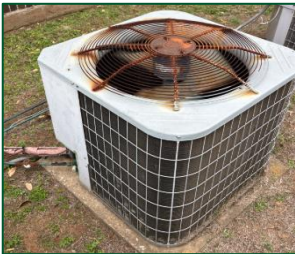
End-of-life condensing units & equipment (20+ years old)
