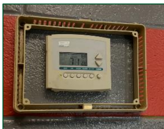
Old thermostats with limited BAS capability
