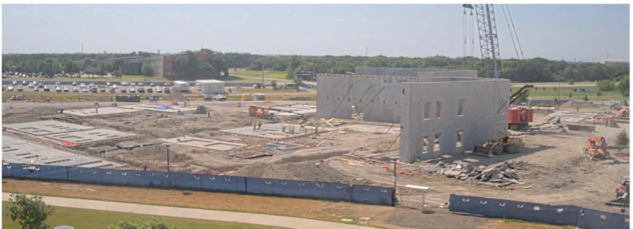
Tilt Wall Panel Erection
