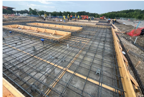
Rebar in Casting Beds
