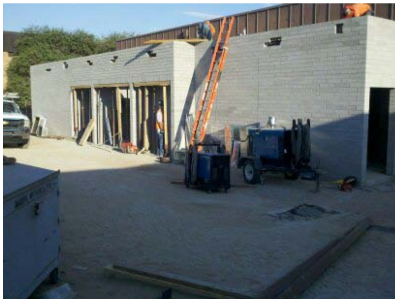
J-3 Restroom Construction
