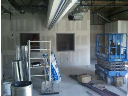
“C” Building IDP Classroom Interior
