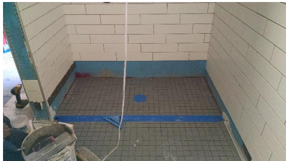
New Shower Area
