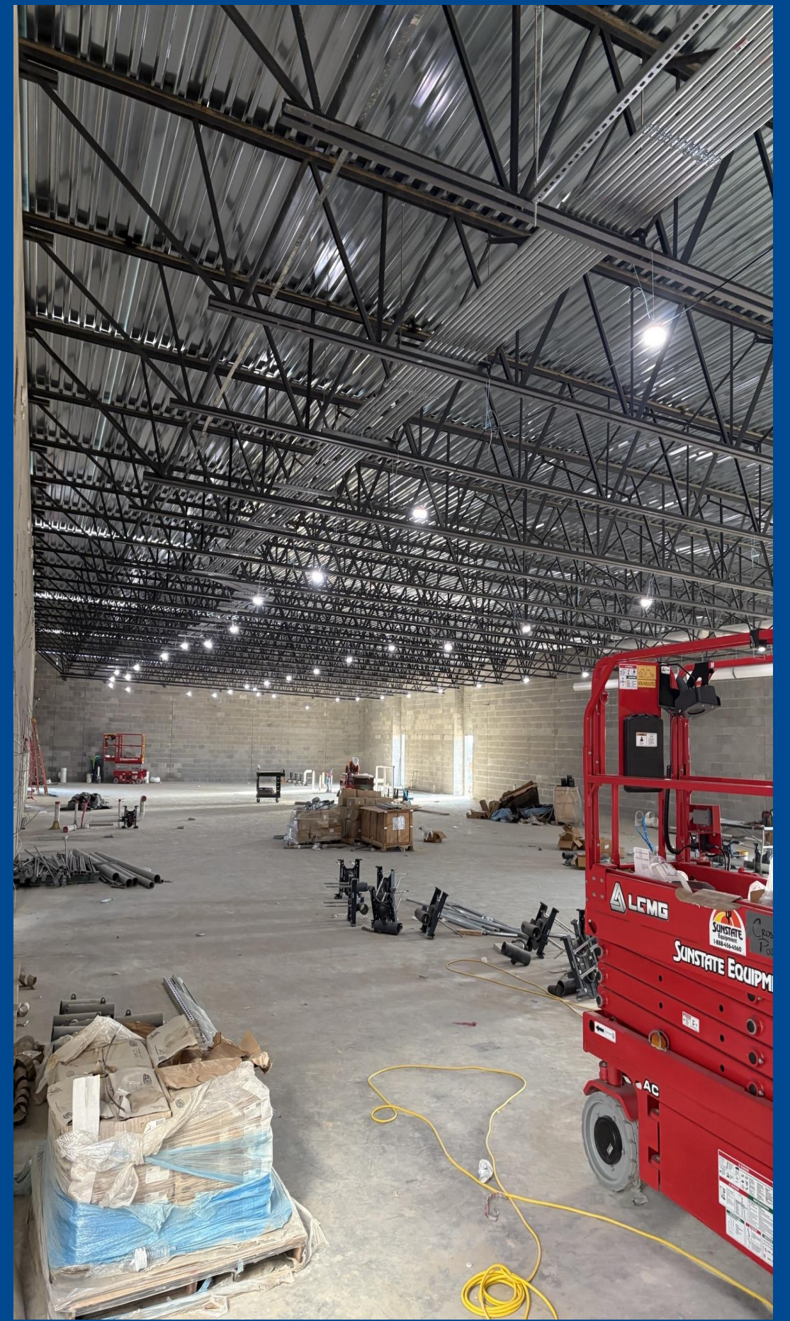
Locker Room Area
