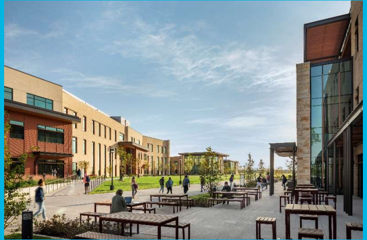
SE View of Campus Quad Area
