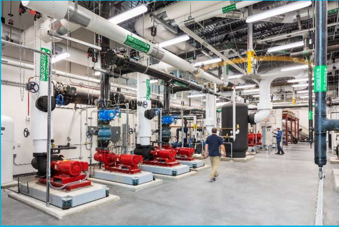
Central Utility Plant
