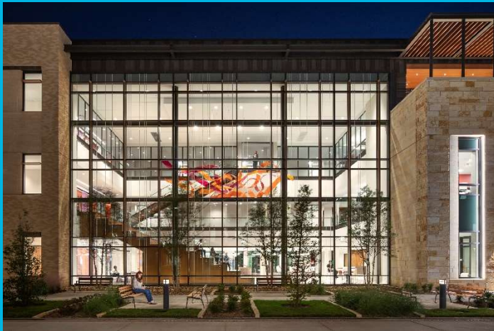
Curtain Wall at Student Center
