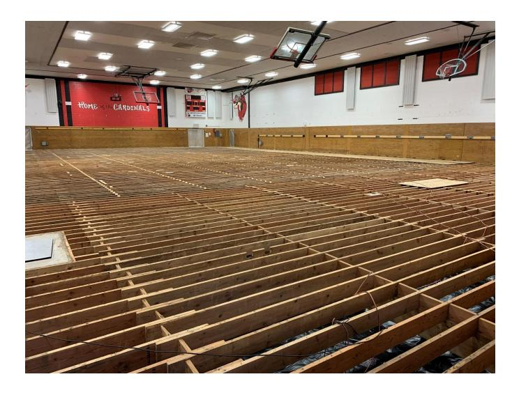
Workers from Flood and Fire Solutions have removed the gym floor, ice blasted the mold from the floor joists, cleaned out the crawl space under the floor, and have put down black visquen over the dirt floor.
