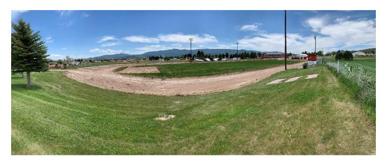
Workers from A+ Contractors have removed the entire base. It was determined the take down the base even further so that the track will be at the same level as the football field. One new long jump runway and pit have been poured.
