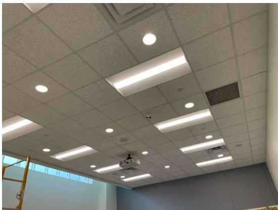
Ceiling Tiles Replaced at Red Room
