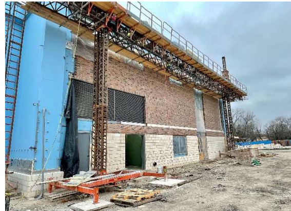
Brick Install on North End of Welcome Center
