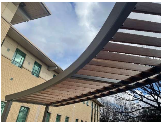
Wood Blades Installed on Trellis at Founders Hall
