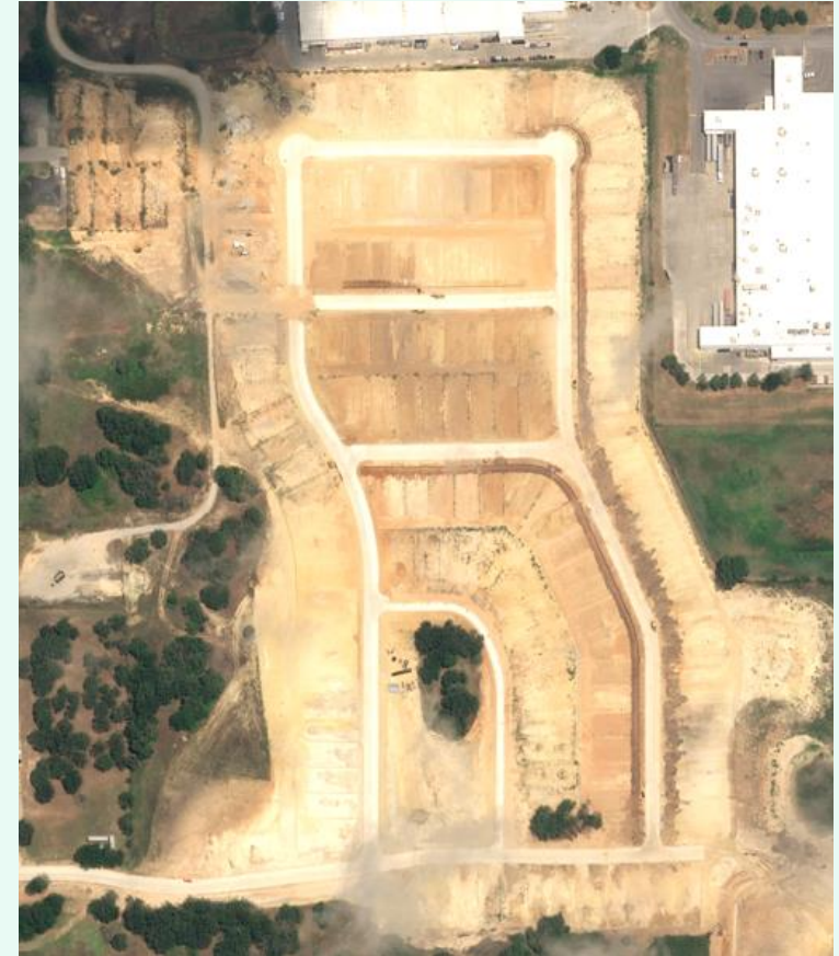
Roads & Utilities Nearly Complete
