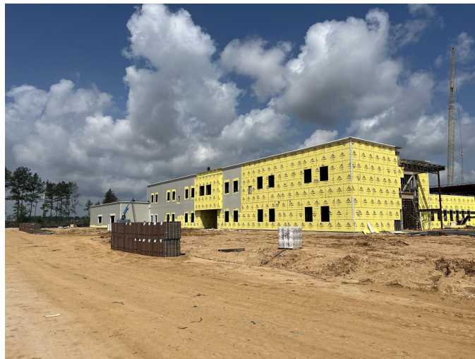
Exterior Waterproofing
