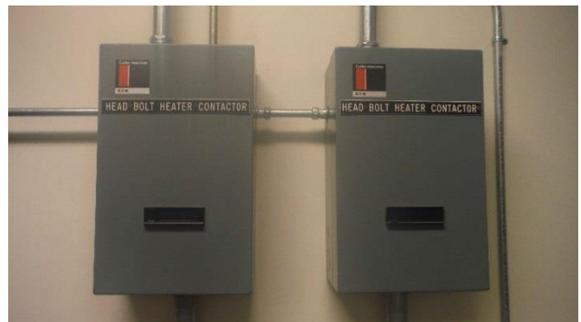
Photo E4– Headbolt Heater Contactors
