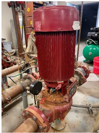
Photo M16– Fire Protection Pump
