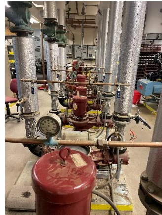
Photo M5 – Heating Pumps
