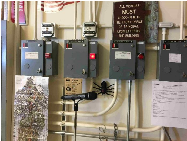
Photo E6– Lighting Contactors
