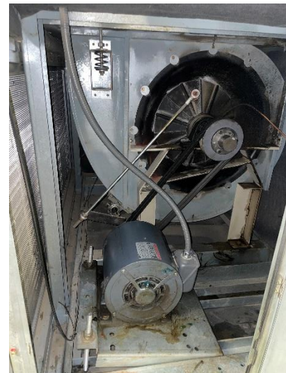
Photo M9 – AHU-5 Inlet Vanes
