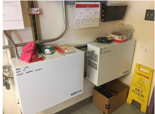
Photo E7– Emergency Lighting Inverters
