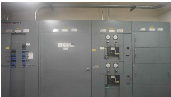
Photo E3– Main Switchgear and ATS
