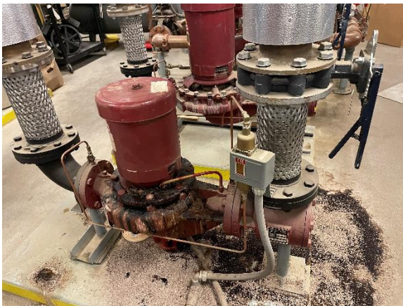
Photo 6 – Leaking Heating Pump
