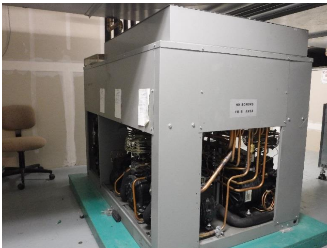
Photo M16- Kitchen condensers located in mezzanine
