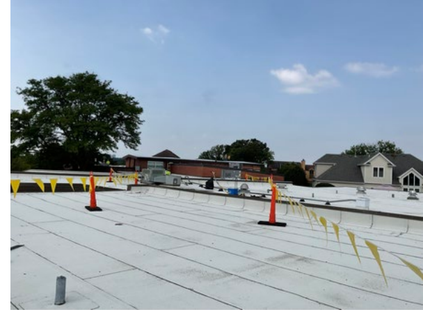
Figure 3: Goodrich New Roofing
