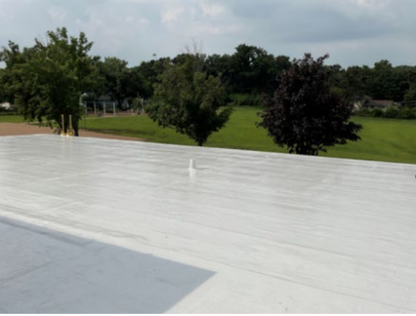
Figure 1: Edgewood Roofing Resurfacing
