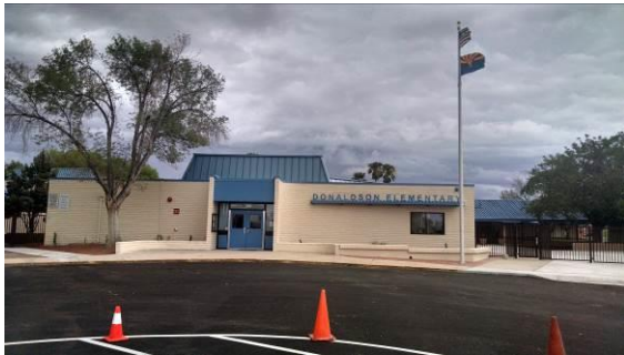
Fresh Paint at Administration
