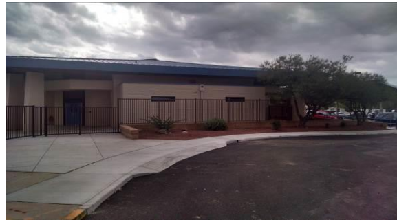
MPR Restroom Addition
