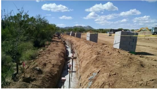
Concrete Footing & Block for West Wall
