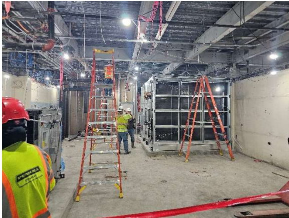
Air Handler moved into place, first floor of H and I of old Science Lab Space
