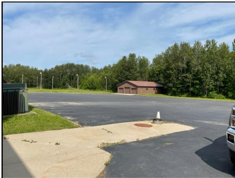
UNDERGROUND FUEL TANK AND STORAGE BLDG
