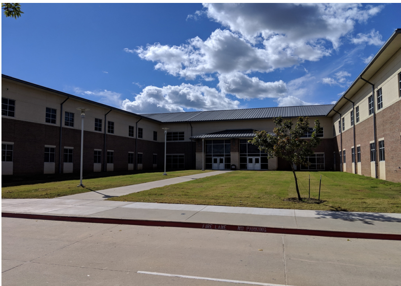
Area B after removal & relocation of portables
