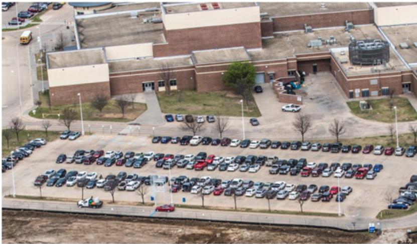
Area D before start of construction
