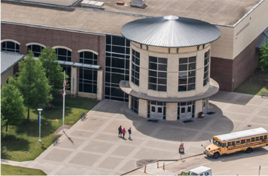
Area A Front Entry Vestibule before start of construction
