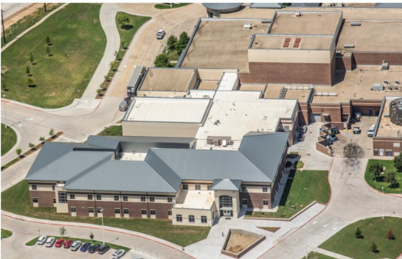
Area D & E Additions/Renovations post construction
