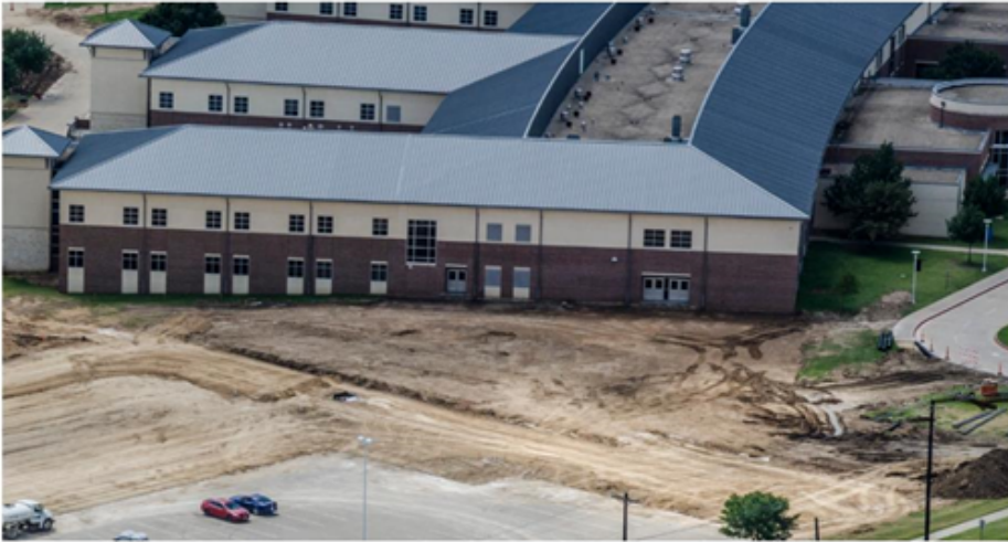
Area C before start of construction
