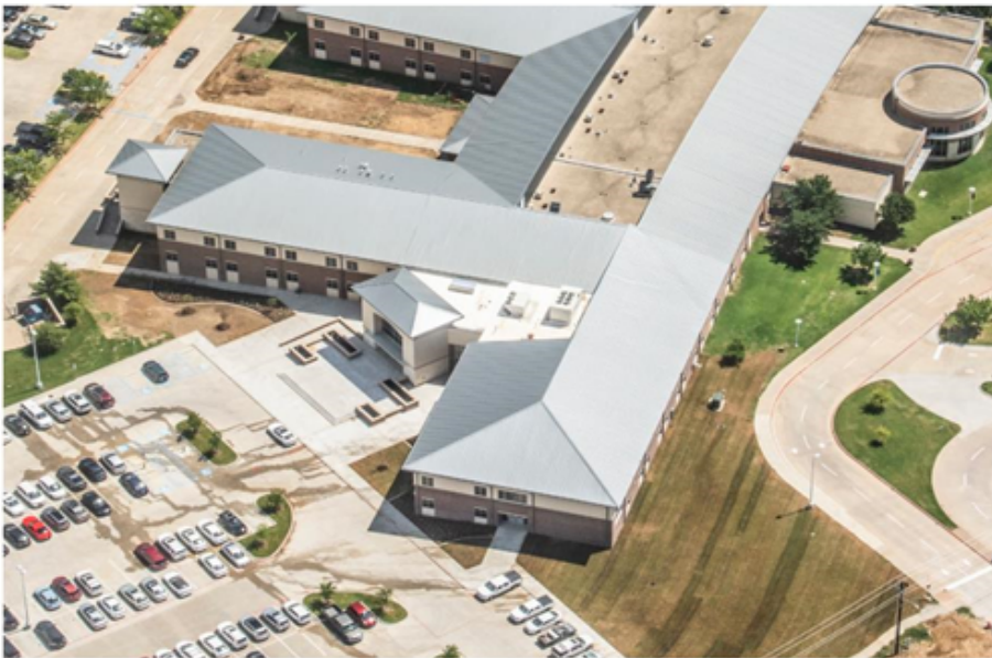
Area C post construction
