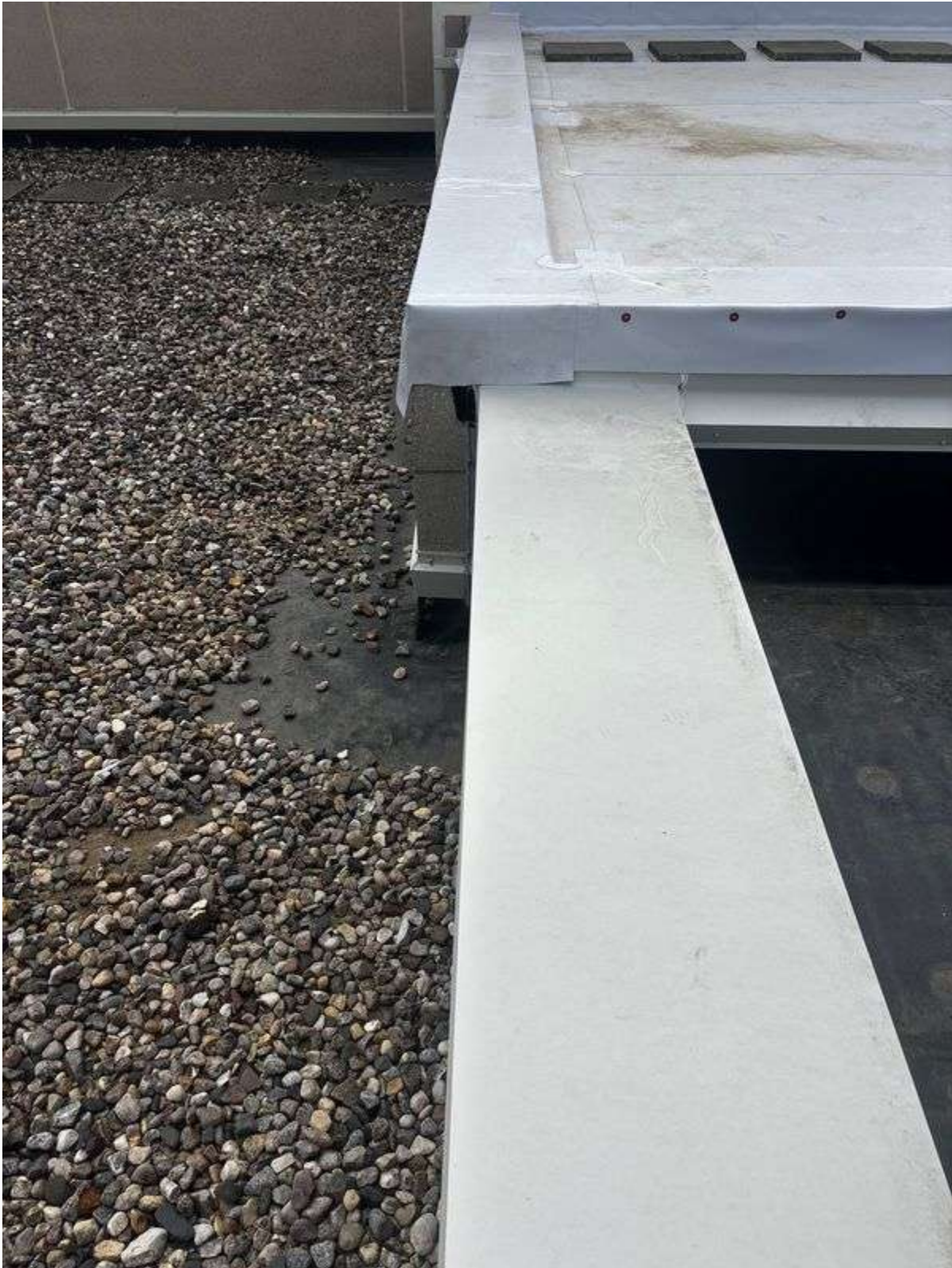
Roof edge detail: heat welded KEE membrane to seal exposed area
