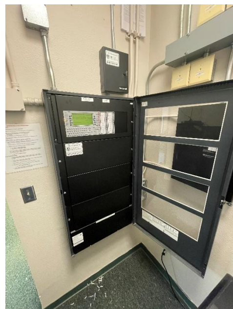
Photo E9– New Fire Alarm Control Panel
