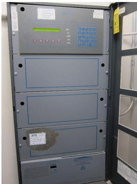
Photo E8– Old Fire Alarm Control Panel
