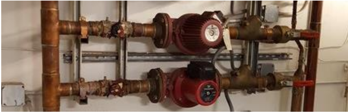
Photo M9 – Typical Elementary School Heating Pumps
