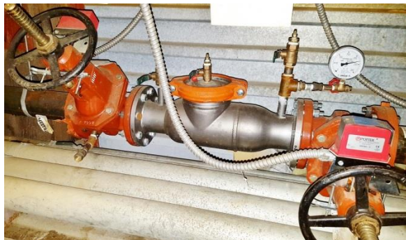
Photo M16 – Vehicle Maint. Double Check Valve
