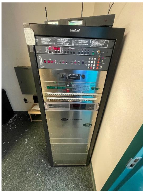
Photo E10 – Intercom Headend Equipment
