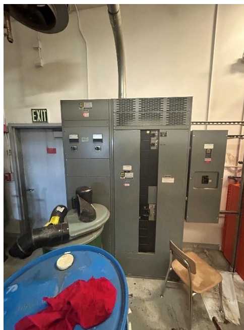
Photo E2– Service Entrance Switchgear
