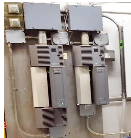
Photo M15 – Typ. MetaSys Controllers
