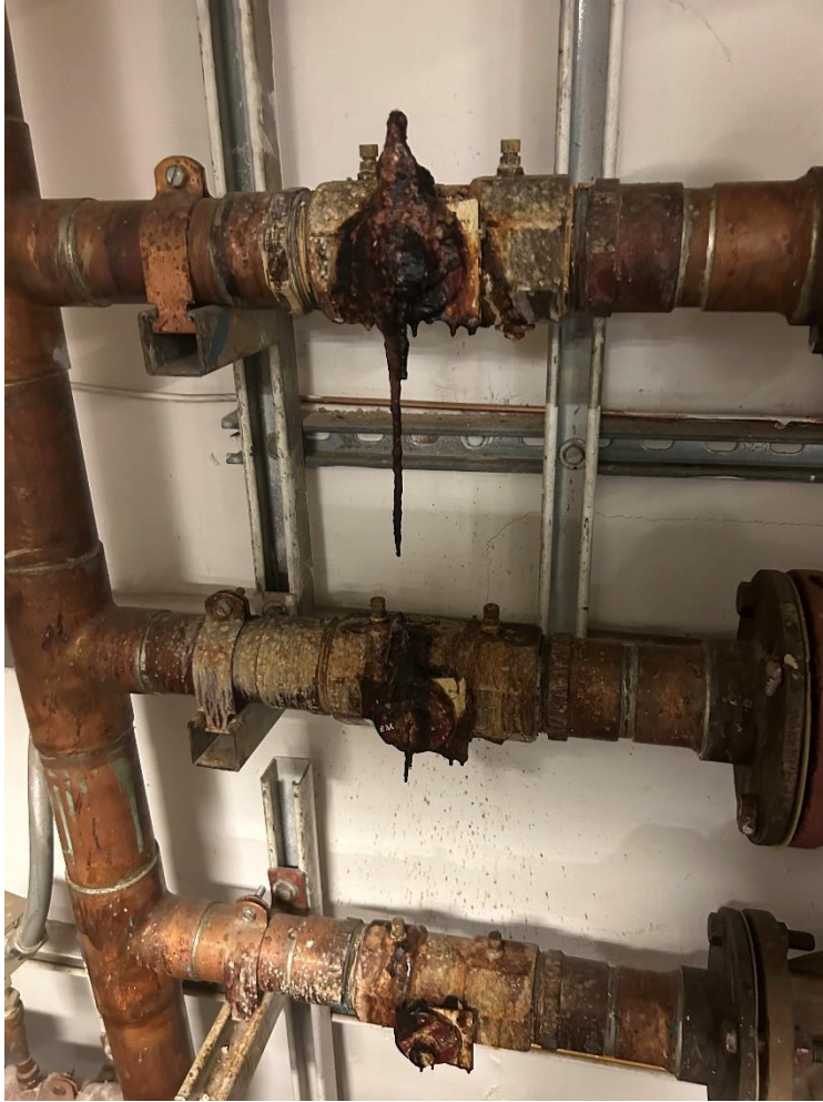
Photo M12 – Glycol Leak at Elementary school circulation pumps
