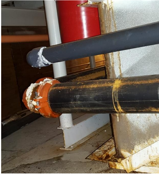
Photo M3 – Leaking and Corrosion Under Pool
