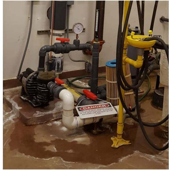
Photo M4 – Leaking Pool Circulation Pump
