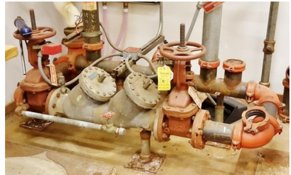
Photo M17 – Pool Mech. Double Check Valve
