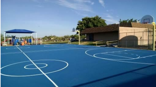
Resurfaced basketball court
