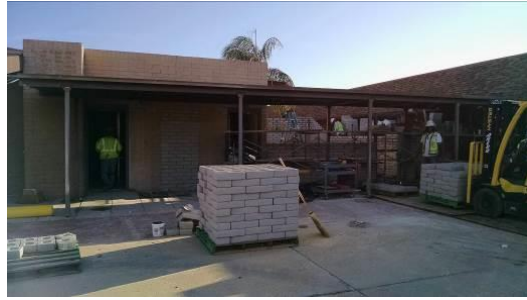
Library restroom renovation
