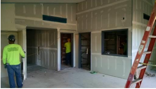
Drywall in the new admin area
