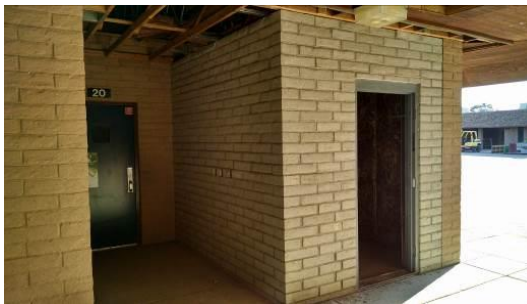
New IDF room addition
