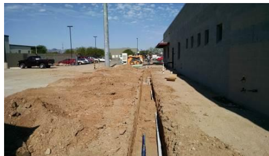
Trenching for water line
