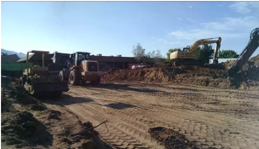
Excavation for new classroom building
