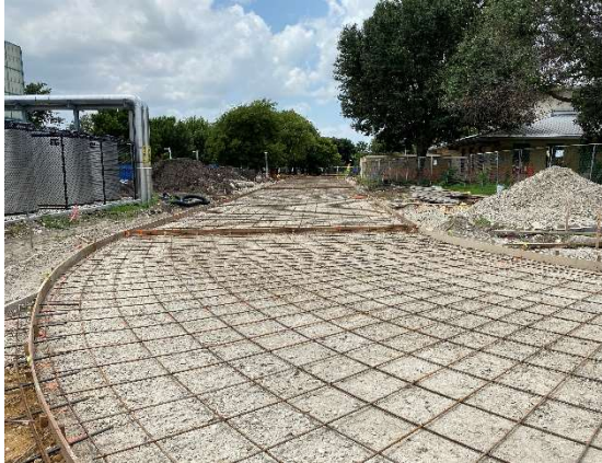
Form and Rebar for Fire Lane
