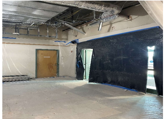
Lobby Entrance at Founder's Hall
