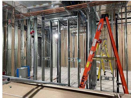
Framing in Dental Area Renovation
