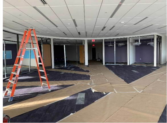
Walls Painted, Light Fixtures and Carpet Installed at Library
