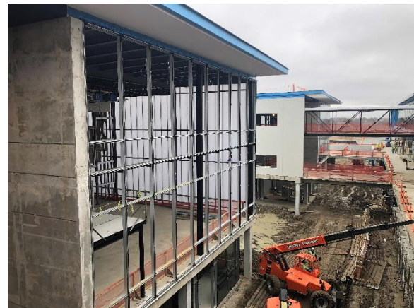
Curtain Wall Framing for Trade Bar C
