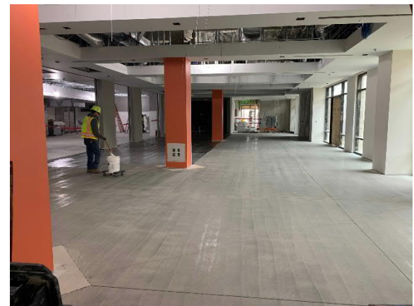
Prepping Floor in the Lobby/Seating Area at Student Center
