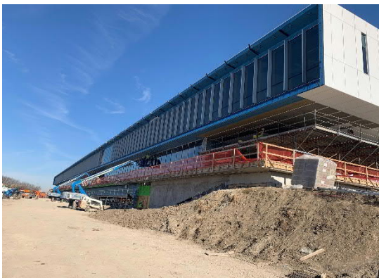
West Elevation of Academic Building
