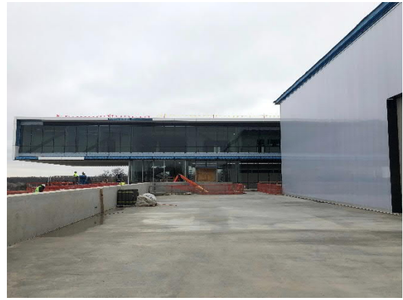
South Overhang of Academic Building
