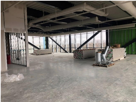
Library on Level 3, North End of Academic Building
