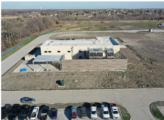
Central Utility Plant
