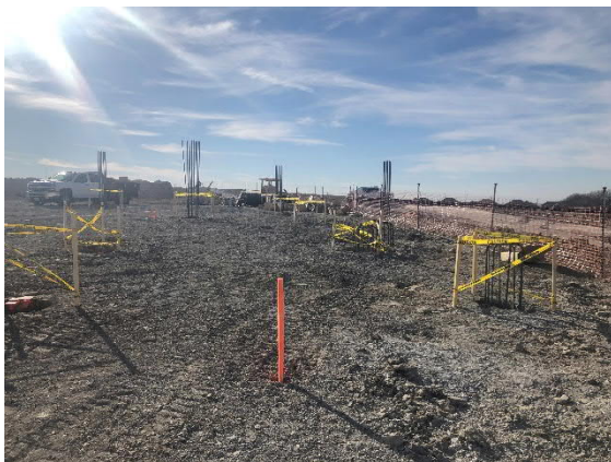
Piers Installed at Building Pad
