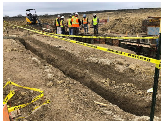
Trench for Piping
