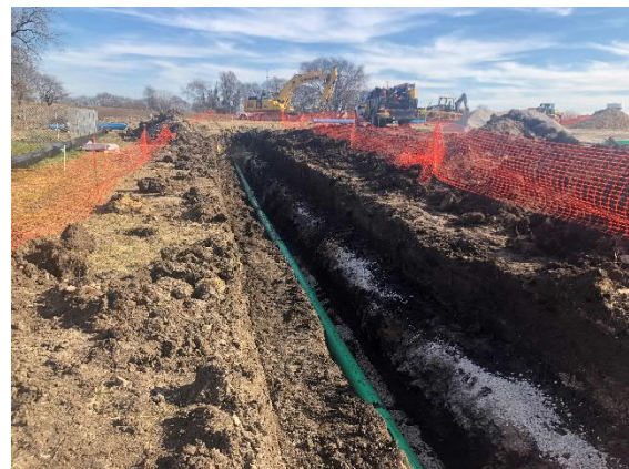
Sanitary Sewer Install
