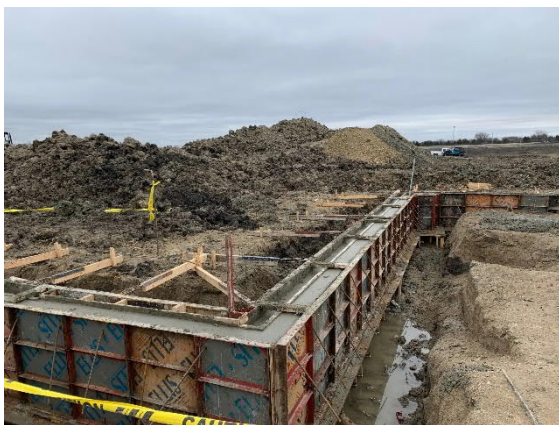
Grade Beams in Area C Poured
