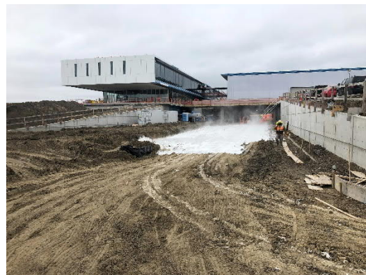
Re-Liming at Garage South Entrance
