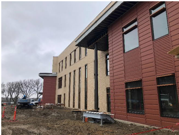
Outdoor Painted Metal Panels at Campus Commons
