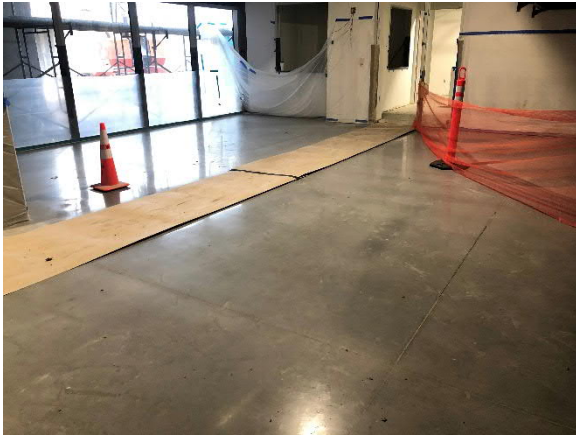
Polished Concrete on Level 1 of Academic Building
