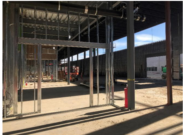
Wall Framing on Level 1 of Trade Bar D
