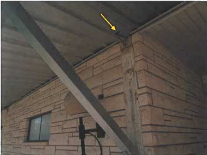
Rust accumulation on structural metal. Trim should be installed over angled protrusions.
