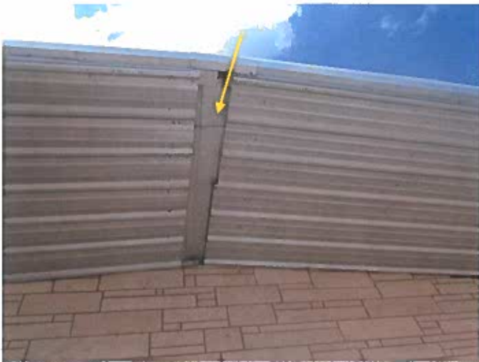
Soffit trim installed without trim closure.
