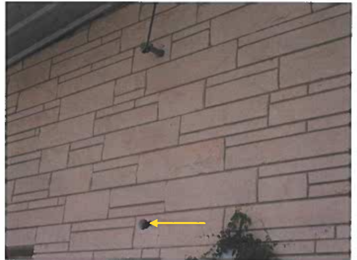
Open wall penetration.
