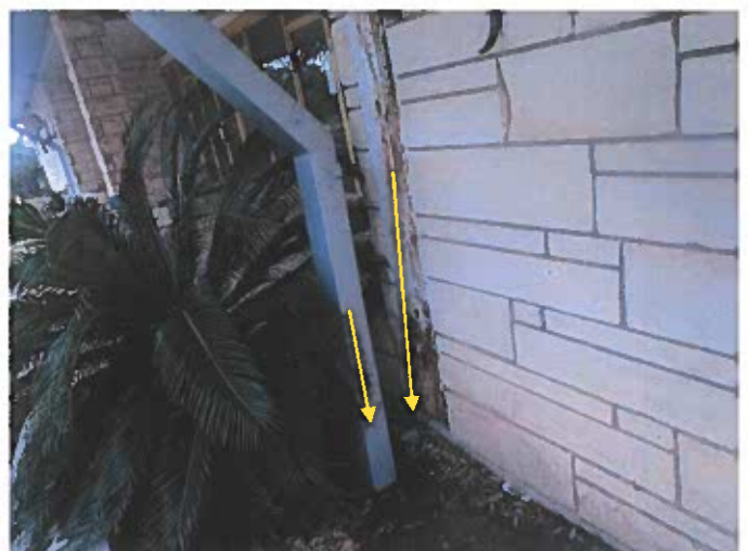
Loose downspout not in drain location.
