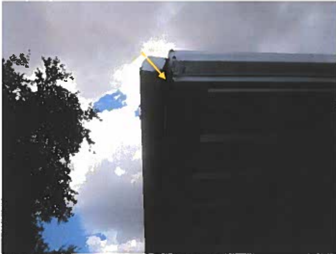
Gutter pulling away from perimeter edge.
