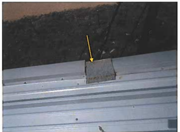
Improper flashing.
