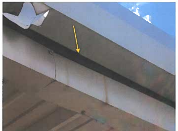
Exposed structural metal.
