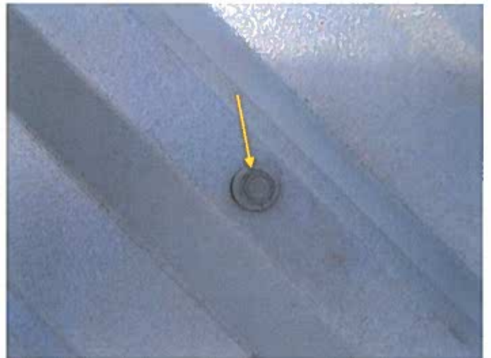
Not a lifetime fastener. Fasteners used of a lower quality than recommended.
