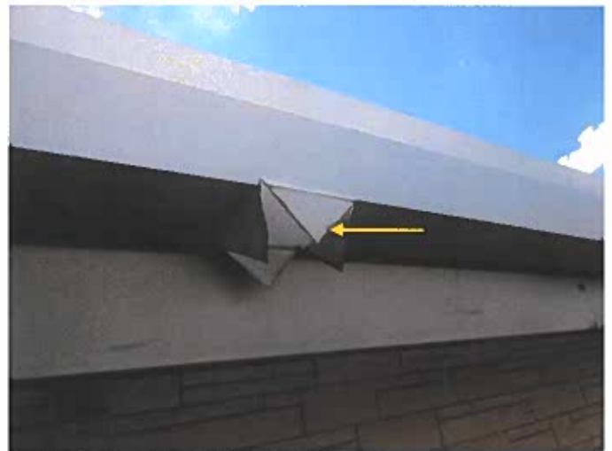
Incomplete and missing downspouts.
