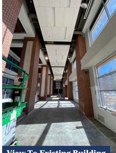
View To Existing Building
