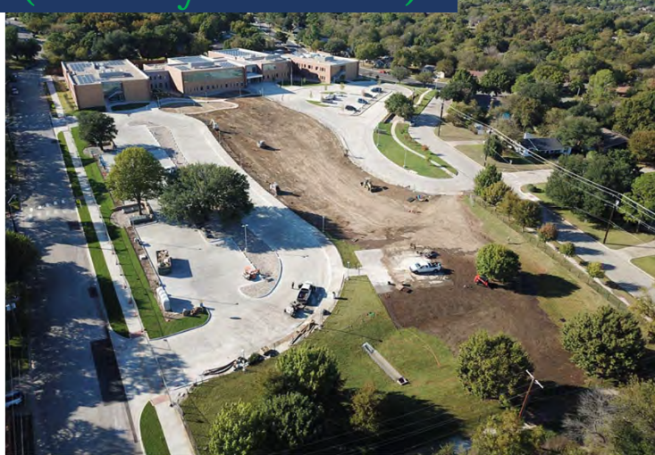
OCTOBER SITE PROGRESS AERIAL
