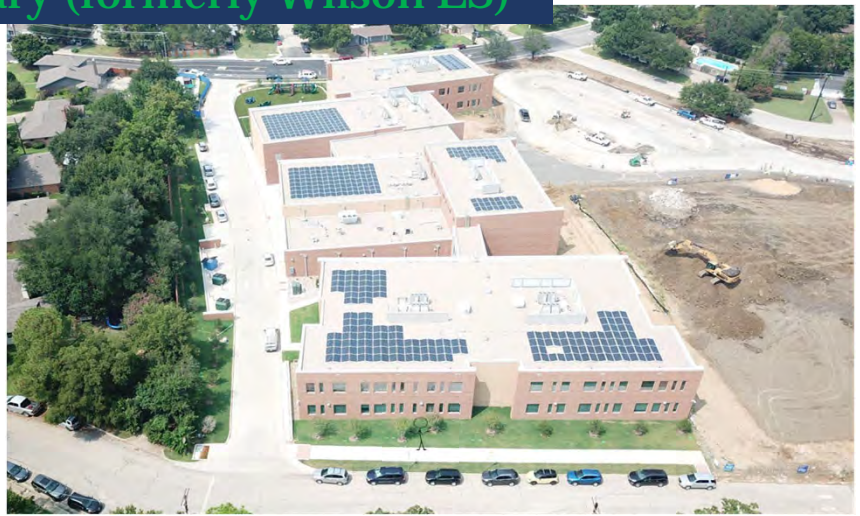
AUGUST SITE PROGRESS AERIAL
