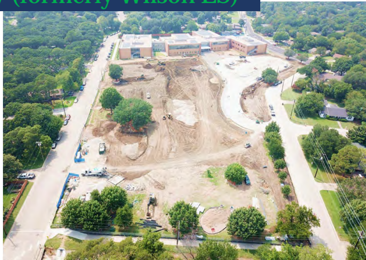
AUGUST SITE PROGRESS AERIAL
