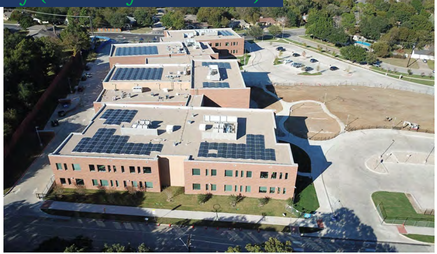
AUGUST SITE PROGRESS AERIAL
