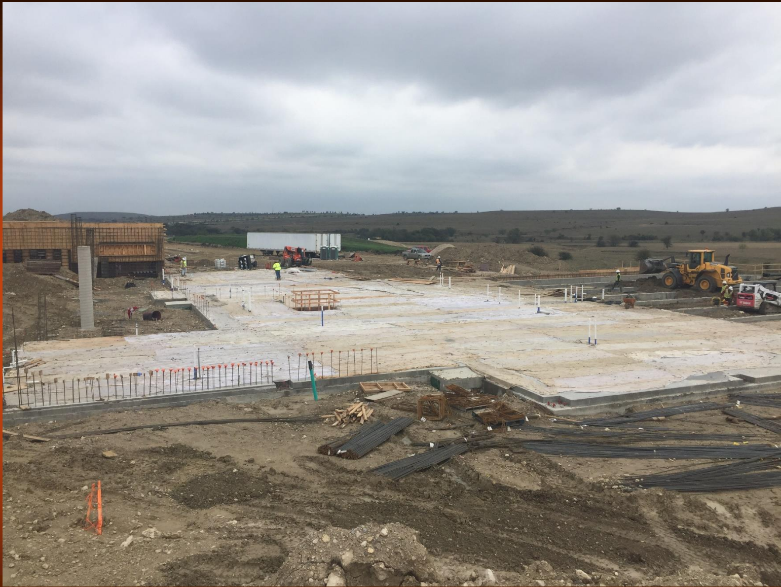
Elementary 5 Area A Slab
