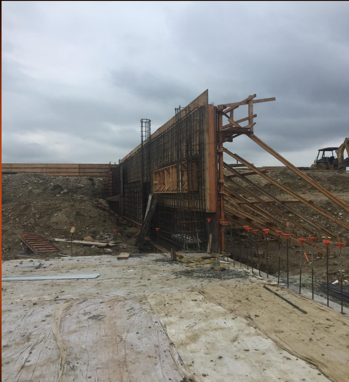
Elementary 5 Grade Beam at Crawlspace Area B
