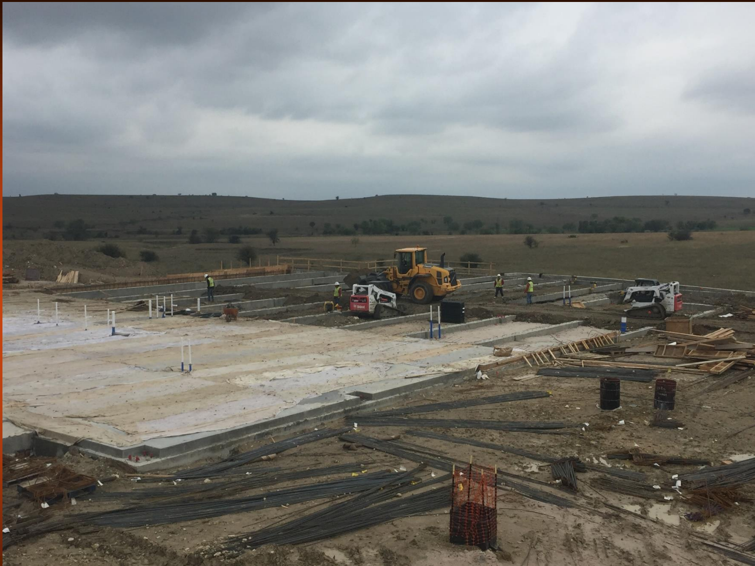
Elementary 5 Backfilling Grade Beams
