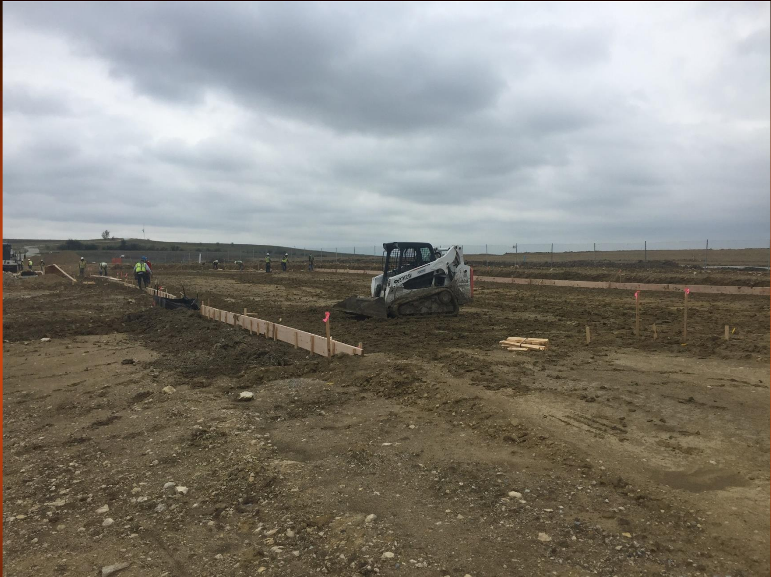
Elementary 5 Installing Forms at North Paving Area
