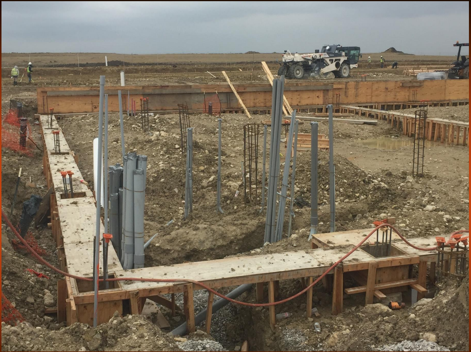
Elementary 5 Electrical Rough-In at Main Electrical Room
