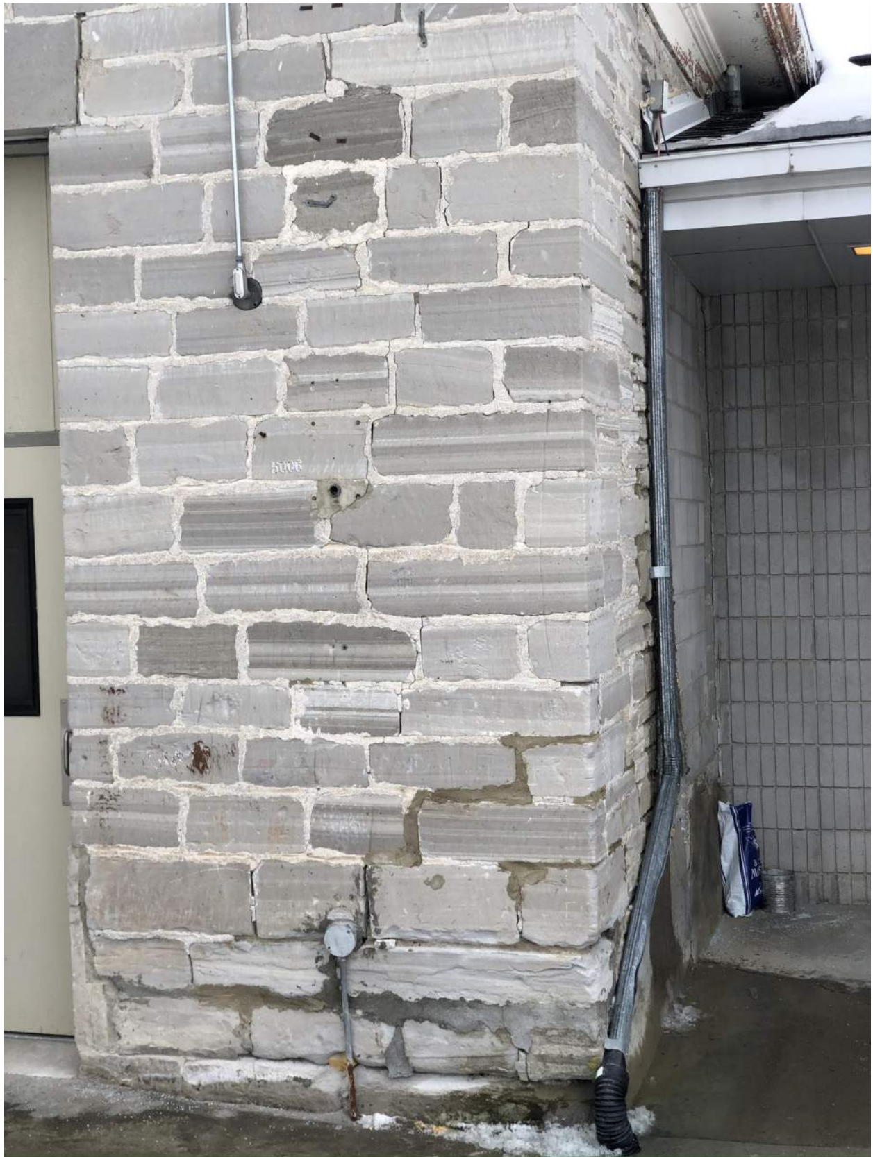
Photo 18 – View of the northwest corner of the kitchen area, near the breezeway. Note mortar deterioration and cracking.
