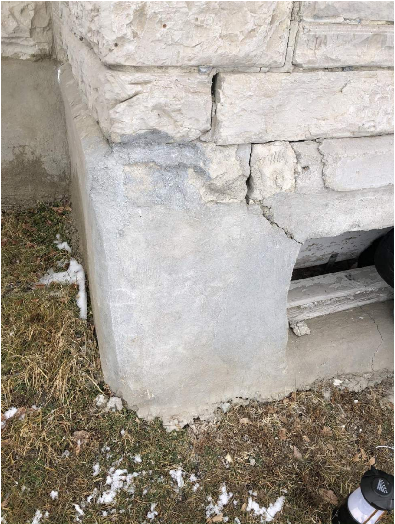
Photo 13 – View of foundation along the south wall. Settlement and cracking are present.
