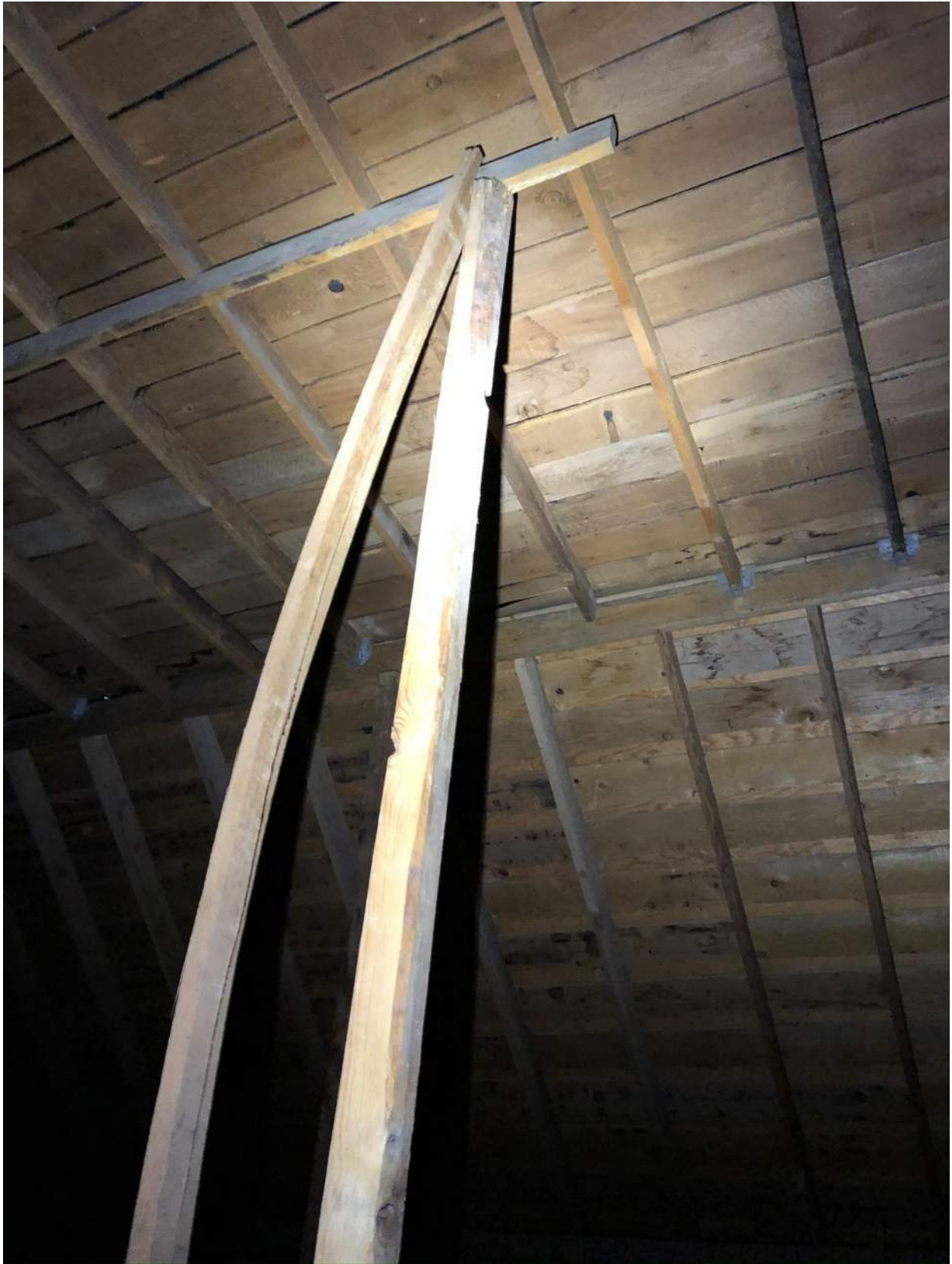
Photo 5 - Existing roof framing over classroom area. Note buckled and bowed bracing member.
